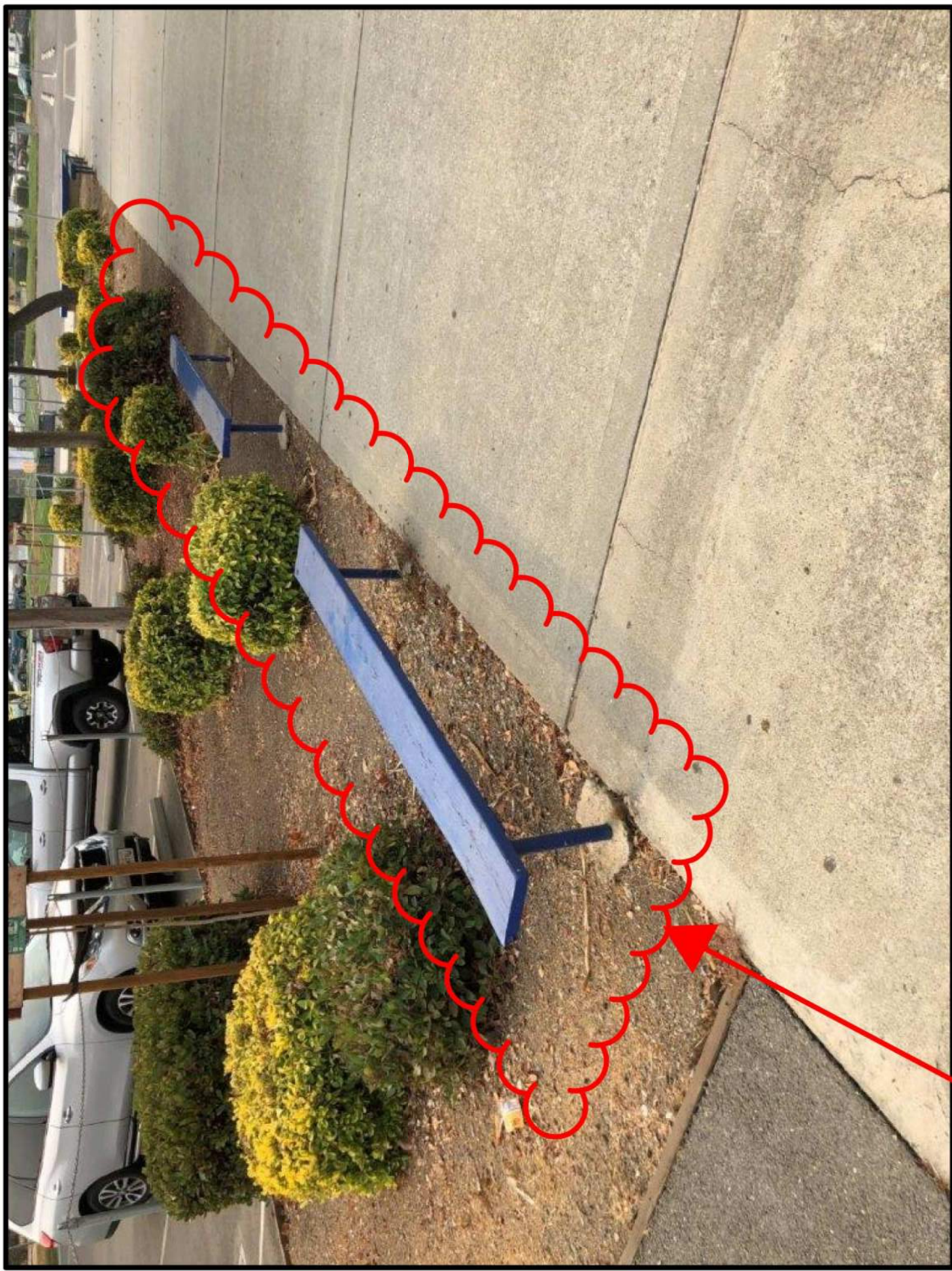
Photo 7: Quantity two (2) existing benches to be removed. Remove bench footing and backfill.
